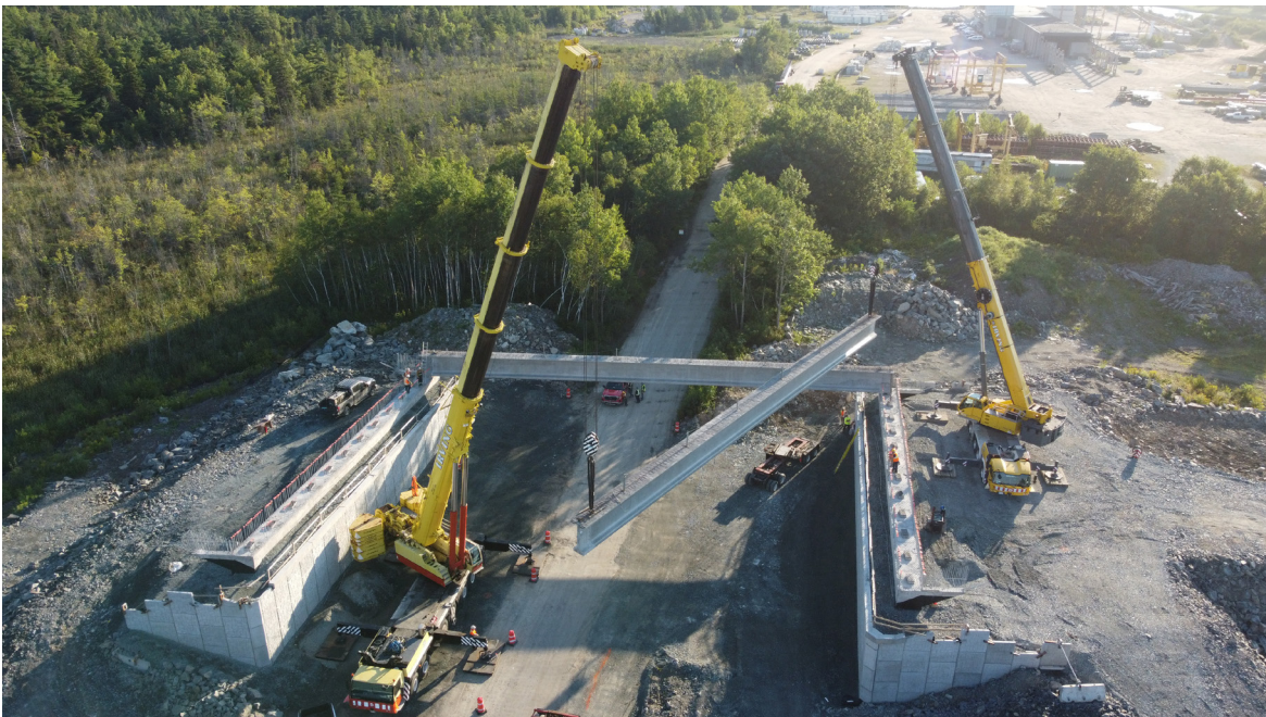
Hwy 107 – Drysdale Ave Overpass
