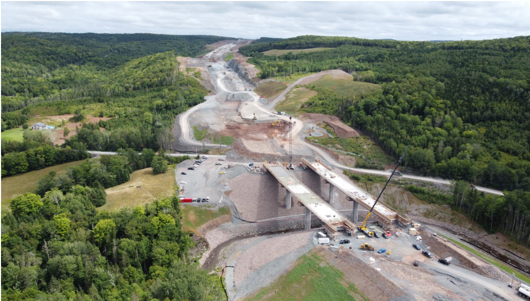
Hwy 104 Middle Brook Bridges
